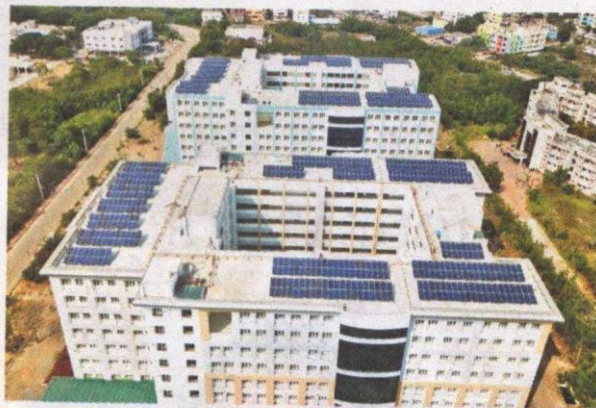
GREEN POWER: The company set up its largest project under Solar Energy Corporation of India at NIT, Warangal.
