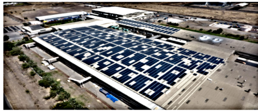
Fourth Partner Energy's 1.5 MW rooftop solar project for Ferrero India, Maharashtra
